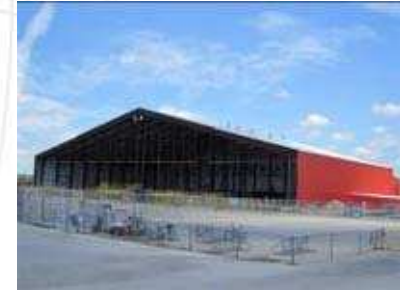
San Antonio new hangar construction
