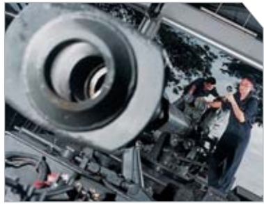
Asset under maintenance
